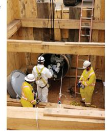
grade changes throughout. Direct access to the infiltration site was not available, so Progressive Pipeline – the general contractor - and the Camden team had to get creative. They created their own pulley system and utilized a body board on wheels to transport their team down the pipe system – 335 feet - which had many angled declines before reaching the infiltration location.
